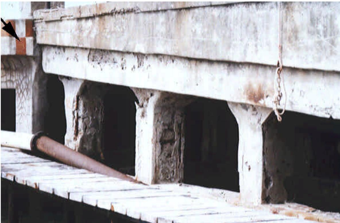
Figure 20 - Crack patterns in a marine structure repaired (on the left) by using high strength shrinkage-compensating mortar.
