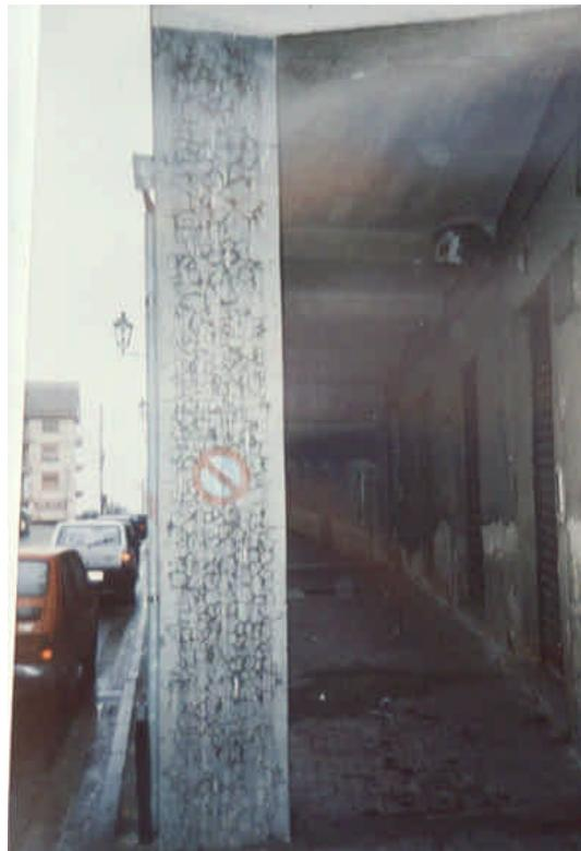
**Figure 24 - Cracked enlargement manufactured with high-strength shrinkage-compensating mortar.**
