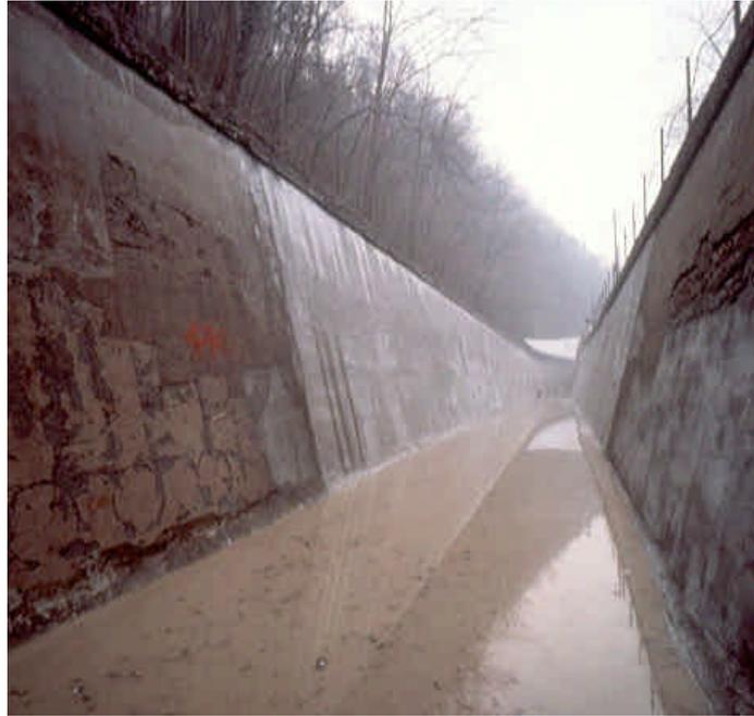
**Figure 23 - Cracks promoted by excessive strain-induced tensile stress from shrinkage in the surface of the cementitious material.**
