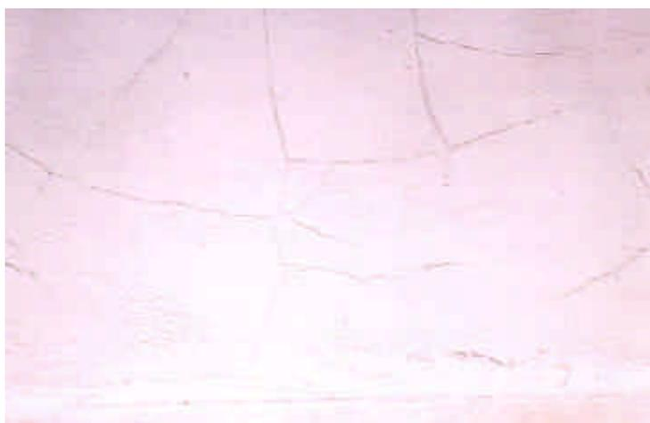
**Figure 22 - Cracks on the surface of the shrinkage-compensating mortar used in repairing cooling tower in Fig. 21.**
