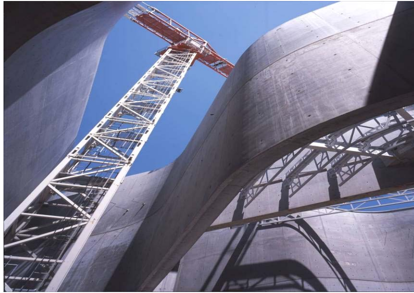
Figure 7 - View of bent and joint-less walls of the MAXXI, Rome, Italy
