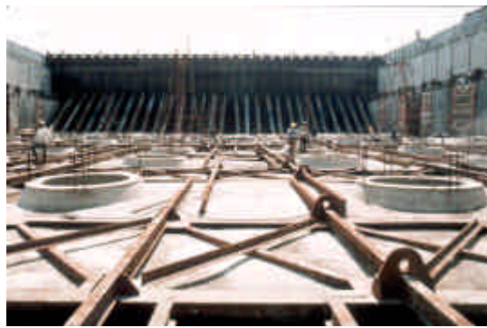
Fig. 5 - View of the reinforced slab foundation placed under water without vibration [4].
