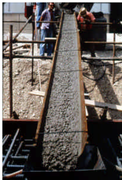
Fig. 6 - Self-compacting concrete placed by chute [8].
