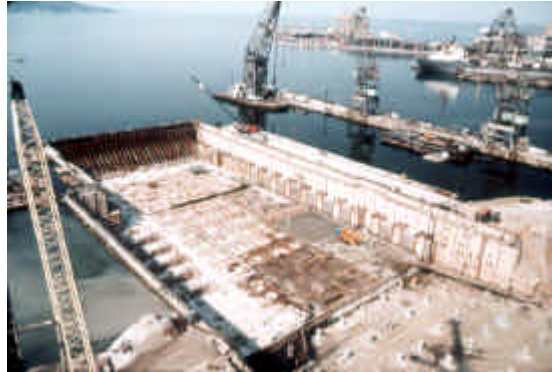
Fig. 4 – Aerial view of the dry dock after removing sea water [4].
