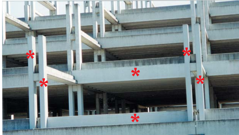
ig. 13.8 – The surfaces with (*) indicate white surface areas due to hydrophobic treatment
