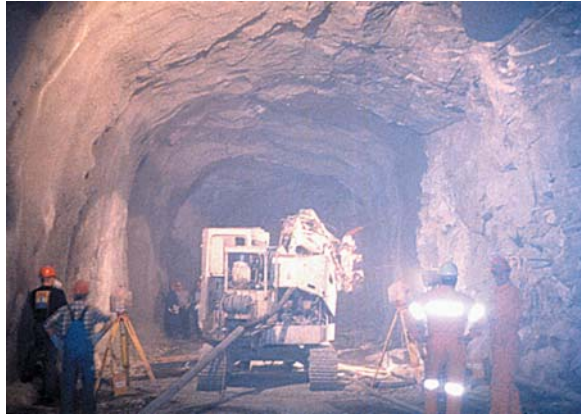
ig. 13.2 – Application of a set-accelerated sprayed concrete in a tunnel
